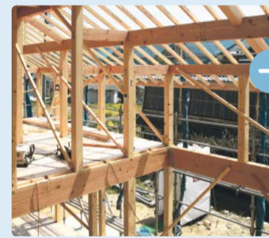
Foto: Pin-connected post and beam house framing, lizenziert unter CC BY 3.0
